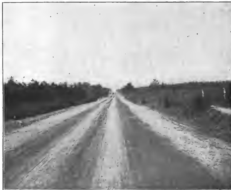
CORLISS AVENUE AFTER IMPROVEMENT—A FINE STRAIGHTAWAY STRETCH.
